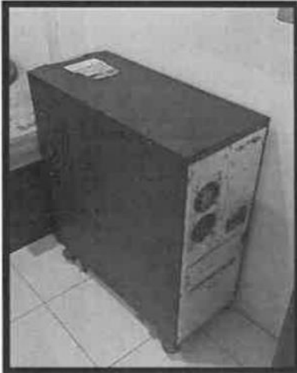
2. KVA UPS W/ Isolation Transformer
