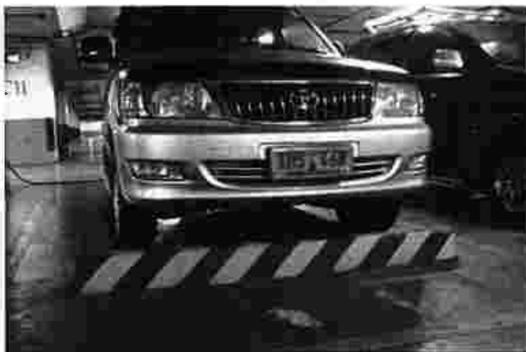
CONCRETE TIRE STOPPER
