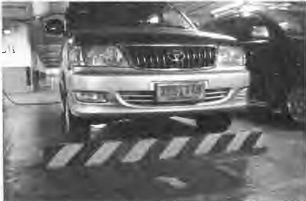
CONCRETE TIRE STOPPER
